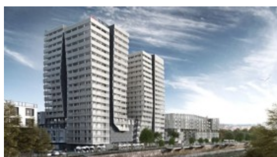
ATAL Towers II / Wrocław
