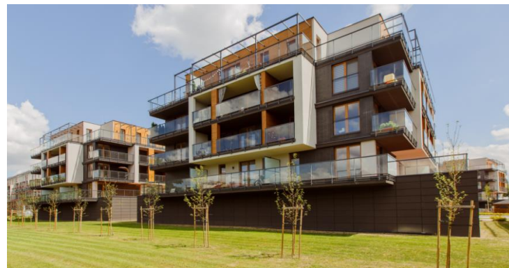
Kraków Bagry Park V (62 lokale)
